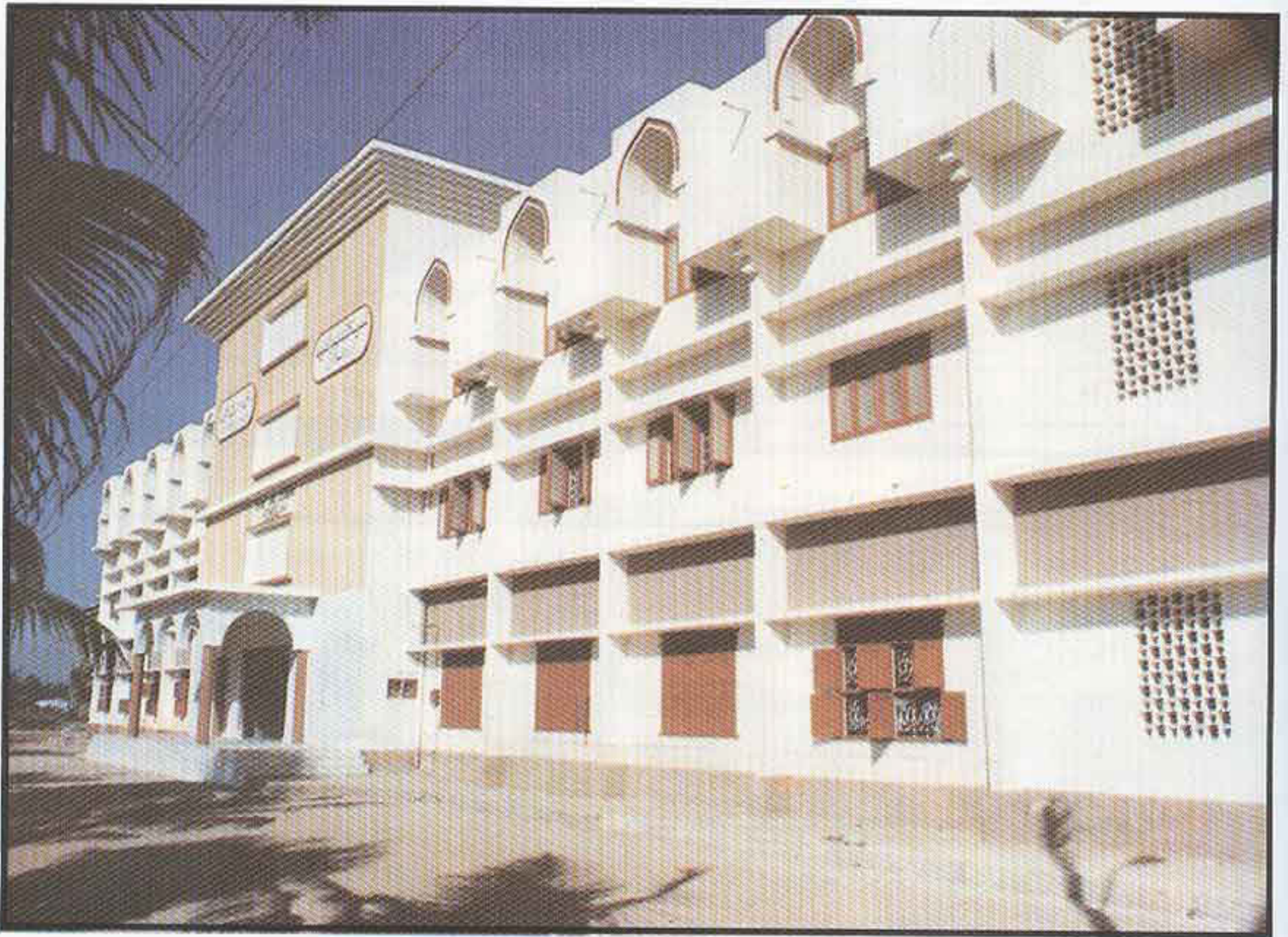
Primary and Secondary School building - front elevation.
